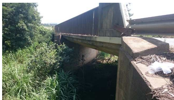
Photo 4. View from the the top of the infilled RHB looking beneath the existing bridge on the Dango River.
